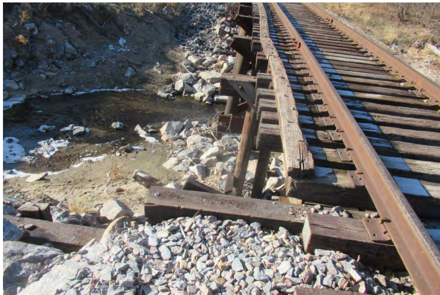
Existing MVRRA bridge over Crow Creek (MP 113.9)
