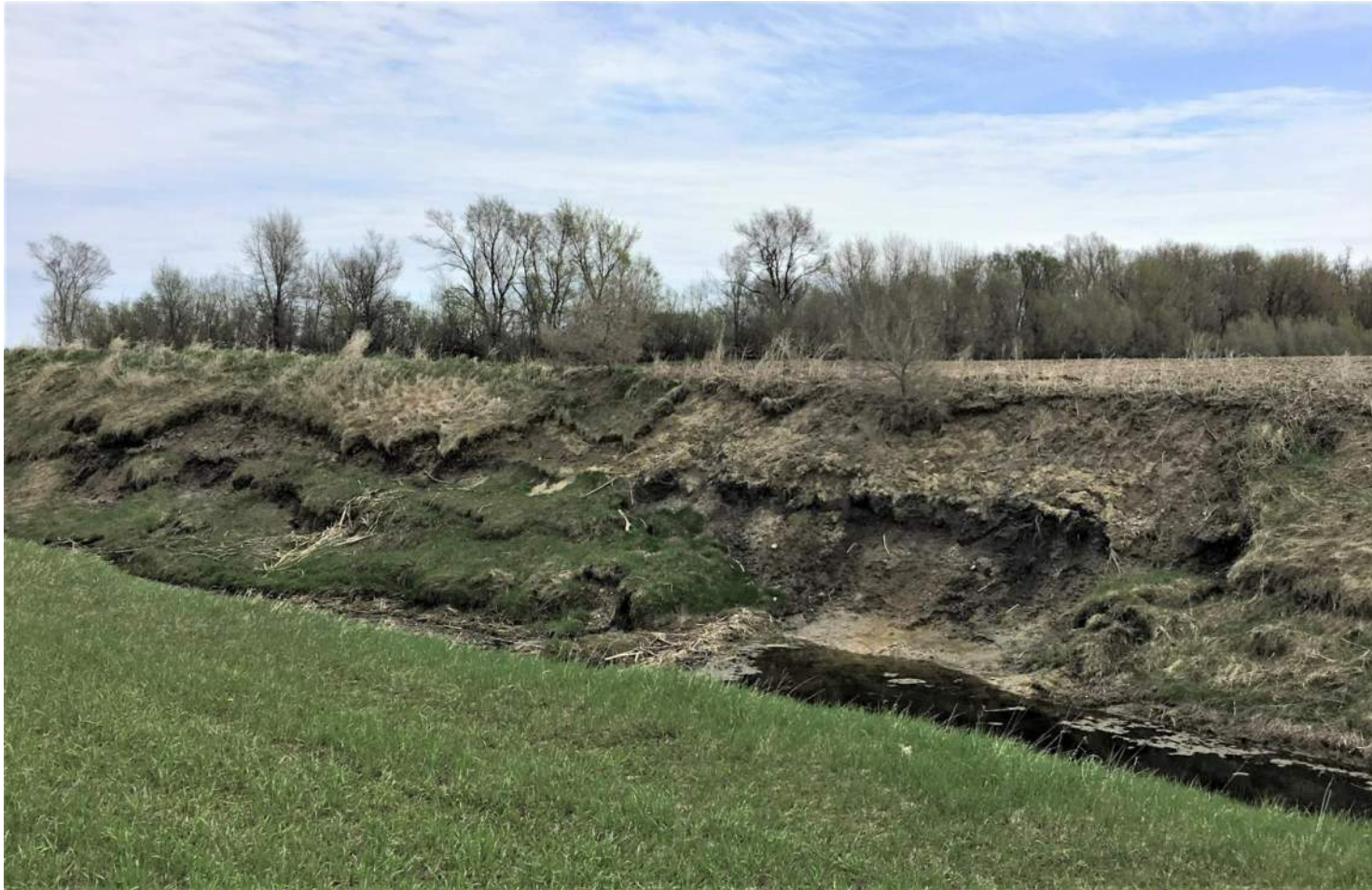
Example of damaged ditch site needing repair
