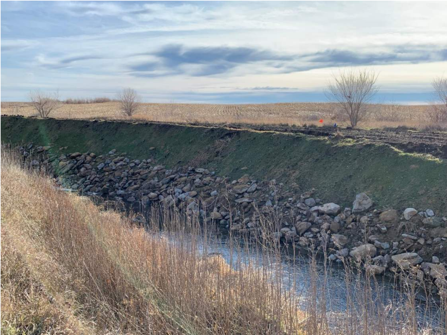
Example of repaired ditch site
