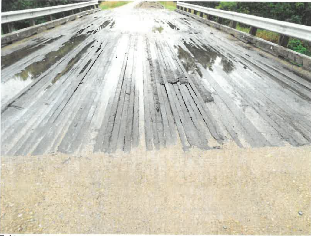
Bridge 64503 bridge deck.
