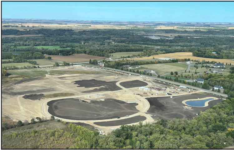
Aerial view of project construction underway
