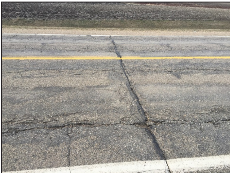
CSAH 13 is planned for pavement rehabilitation in 2023, which will be a mill and overlay project.
