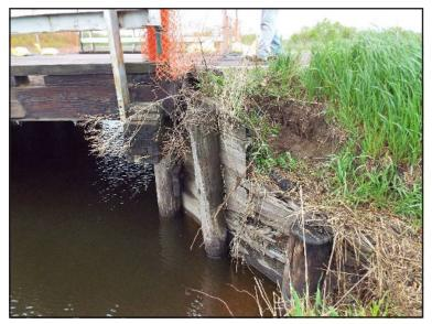
CSAH 8 Bridge 89825 replacement that occurred in September 2022. Note the advanced deterioration of the abutment and abutment pile caps.
