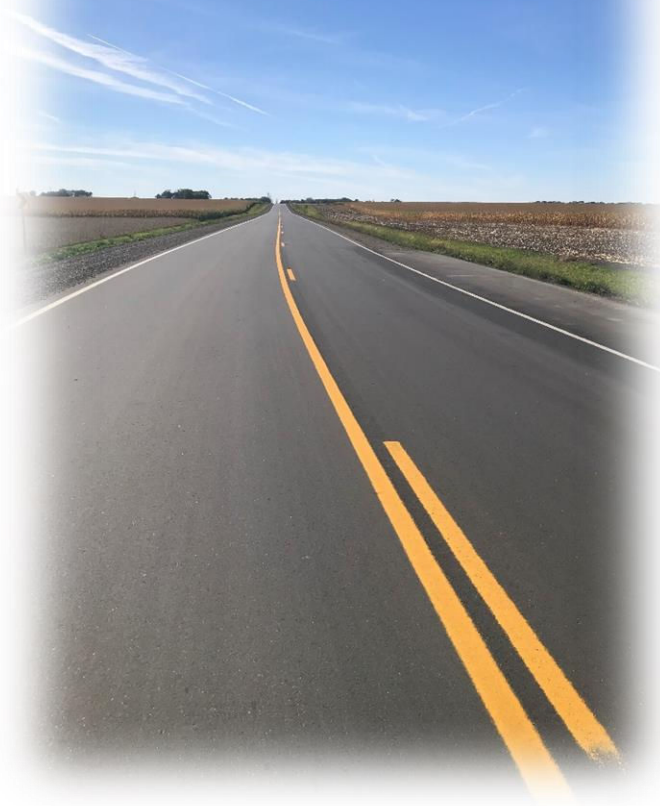
2022 Cold-in-Place Recycling and Paving of CSAH 6 North of Wabasso, MN
