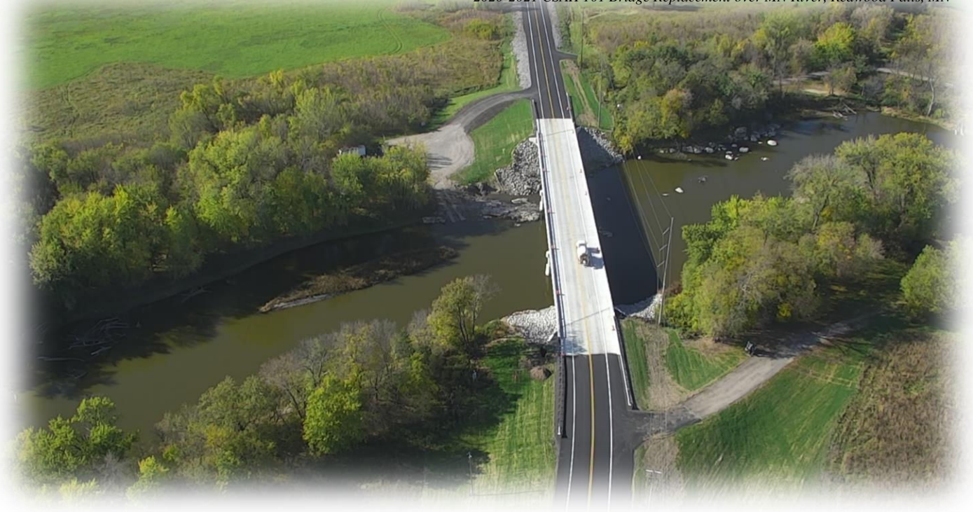
2020-2021 CSAH 101 Bridge Replacement over MN River, Redwood Falls, MN
