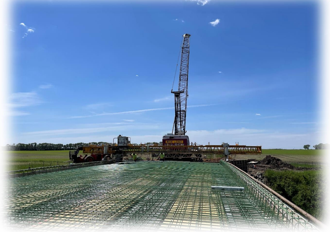
2022 Magnolia Ave Bridge Replacement over Sleepy Eye Creek, Sundown Township MN
