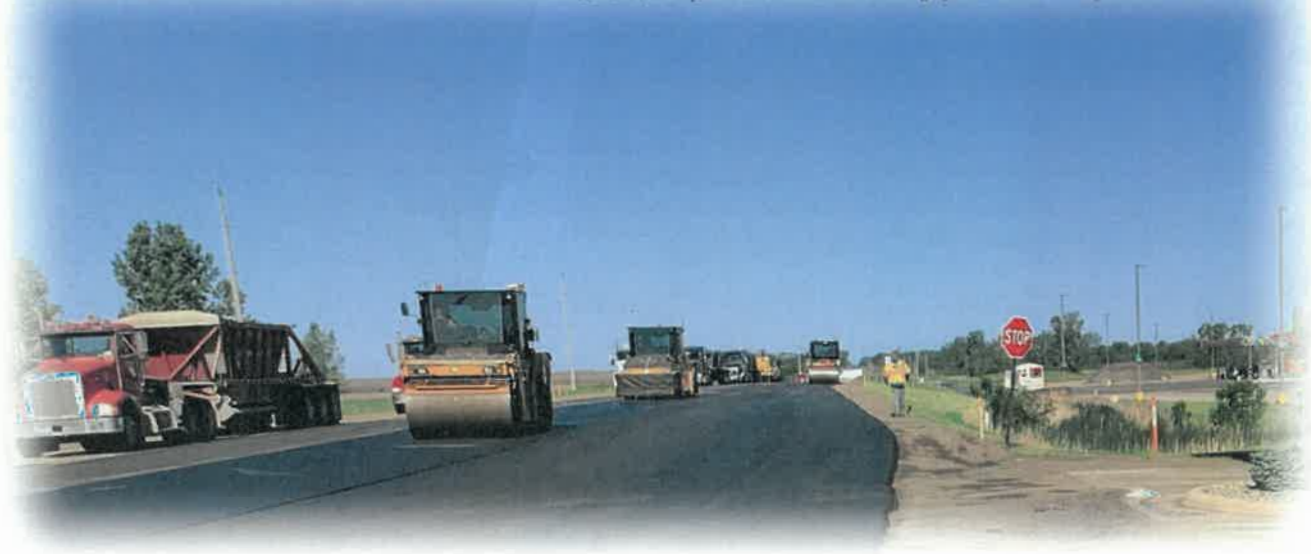
2022 Full Depth Reclamation and Paving of CSAH 24, East of Redwood Falls, MN
