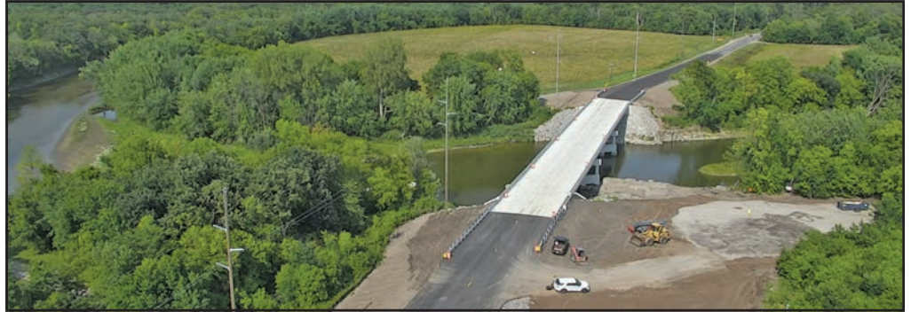
CSAH 101 MN River Bridge on September 2, 2021
