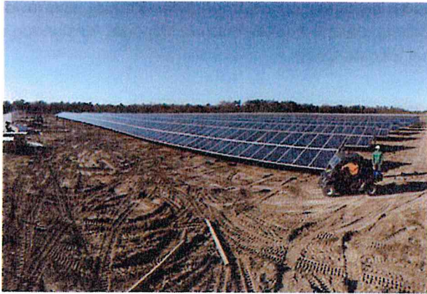
EXAMPLE OF A SOLAR PROJECT IN CONSTRUCTION
