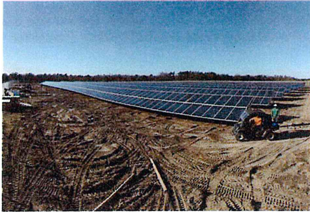
EXAMPLE OF A SOLAR PROJECT IN CONSTRUCTION
