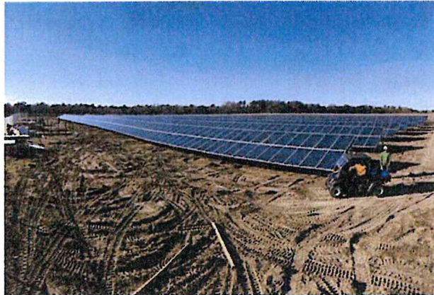
EXAMPLE OF A SOLAR PROJECT IN CONSTRUCTION
