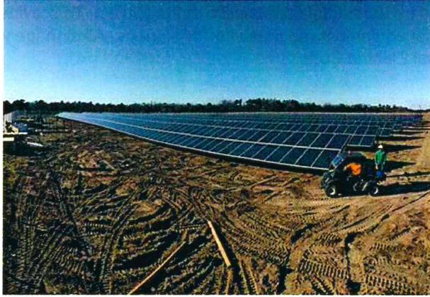
EXAMPLE OF A SOLAR PROJECT IN CONSTRUCTION
