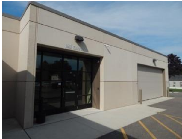
(Main Entrance to the Redwood County Jail)
