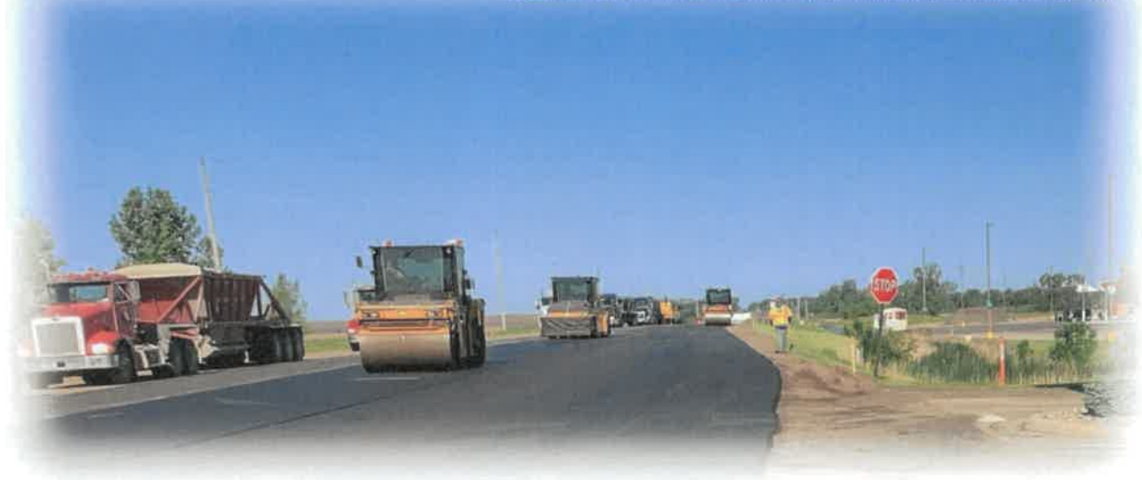
2022 Full Depth Reclamation and Paving of CSAH 24, East of Redwood Falls, MN
