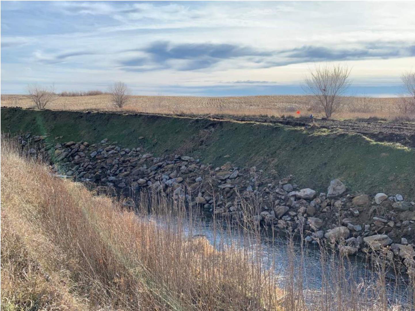
Example of repaired ditch site
