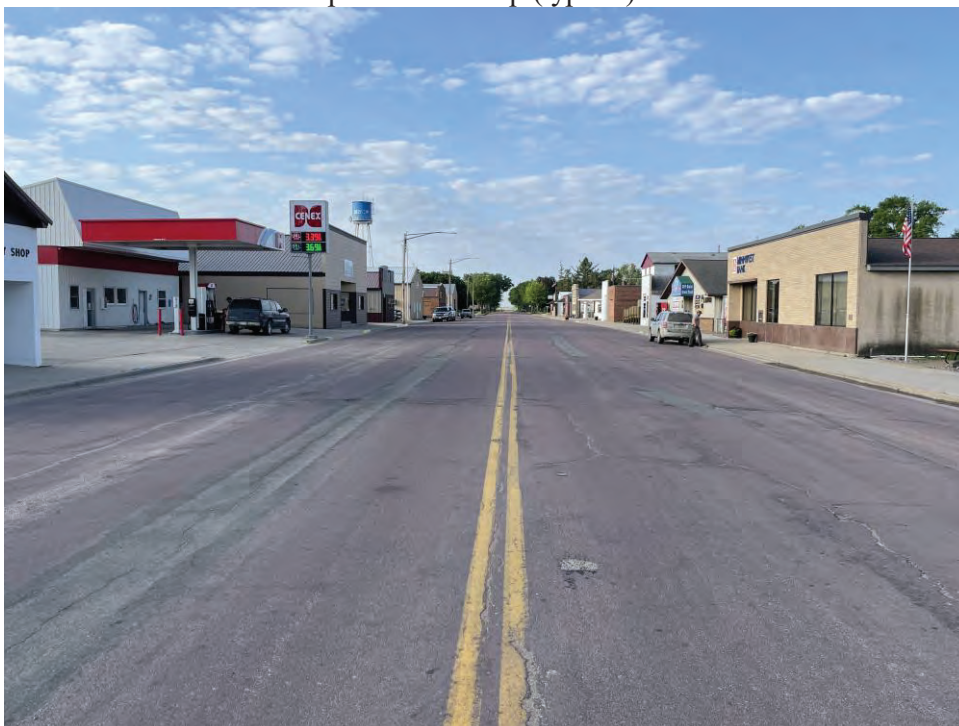
CSAH 7, south of Elevator Avenue, Facing South. Note strong business development and downtown business livelihood, including Minnwest Bank, Cenex Fuel Station, Farmers Grain Elevator, Real Estate Agency, multiple restaurants, Farmers Co-op Electric Company, US Post Office, City Shop, multiple automotive repair shops, multiple churches, etc. Note multiple patches, rutting in tire paths and longitudinal cracking.
